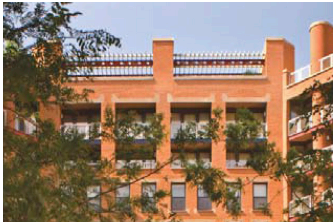
VIEW OF SIMILAR ROOF TOWER FEATURE AT JEFFERSON PENN QUARTER
